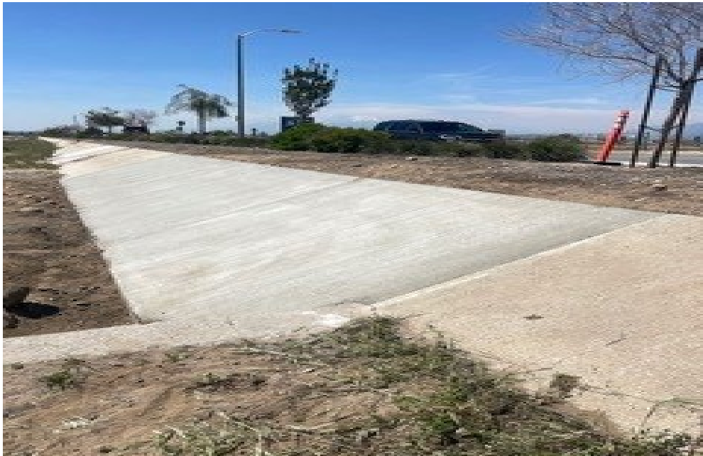
CITY CREEK BYPASS CHANNEL, WALL FAILURE AND UNDERMINE, AREA 1, PRE AND POST REPLACEMENT
