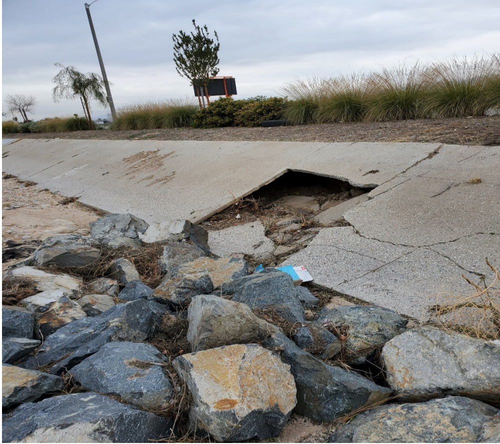
CITY CREEK BYPASS CHANNEL, WALL FAILURE AND UNDERMINE, AREA 1, PRE AND POST REPLACEMENT
