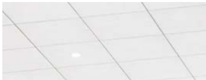
Armstrong Ceiling System White, 24"x24" Existing Ceiling grid to remain New Ceiling tile to match existing
